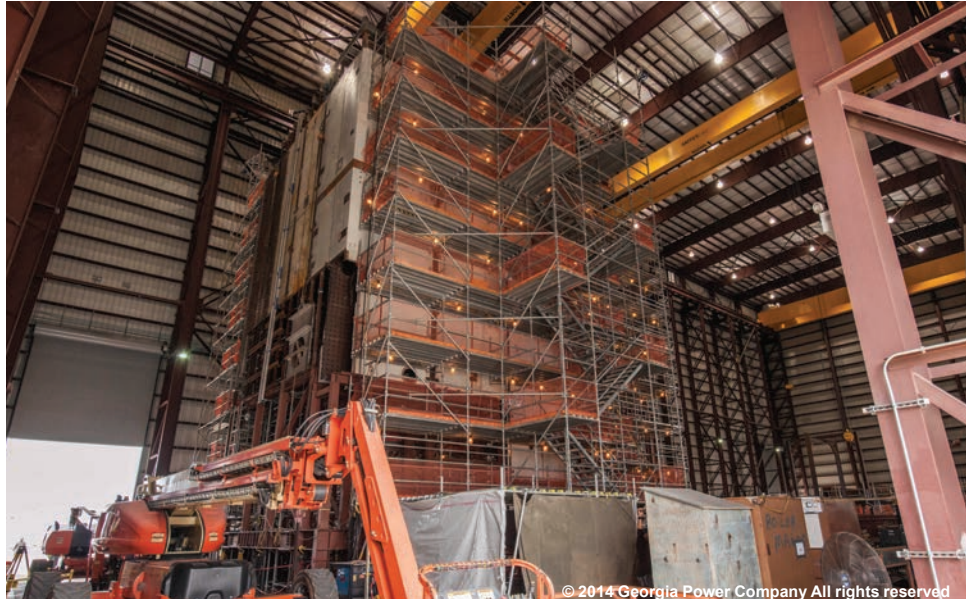
Plant Vogtle Unit 3 CA-01 module inside the module assembly building.
