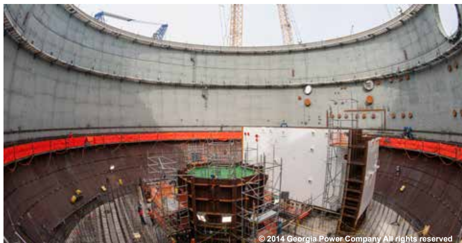
Plant Vogtle Unit 3: CA-04 and CA-05 inside the containment vessel.
