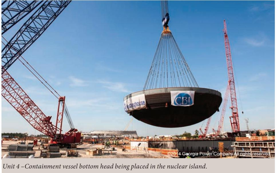
Unit 4 – Containment vessel bottom head being placed in the nuclear island.
